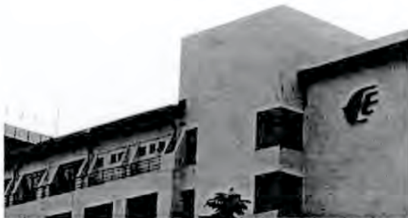
Figure 1. A picture of the Malaysia Airline building taken in 1995 showing the ESE air terminal (left).
