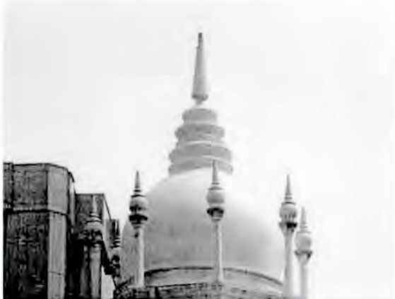
Figure 5. A lightning damaged spire on top of a dome. Note the stricken point below the pinnacle.
